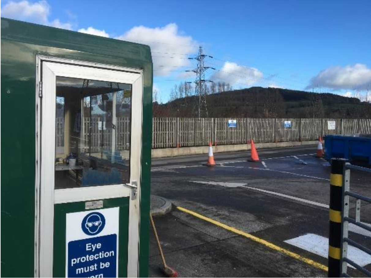
Figure 11: Public Exit from the Llanfoist HWRC (E.How 31/02/2019)
