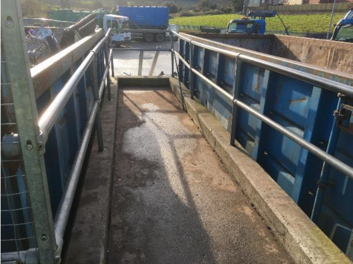
Figure 18: Pedestrian Access to Recycling Containers (E.How 31/02/2019)
