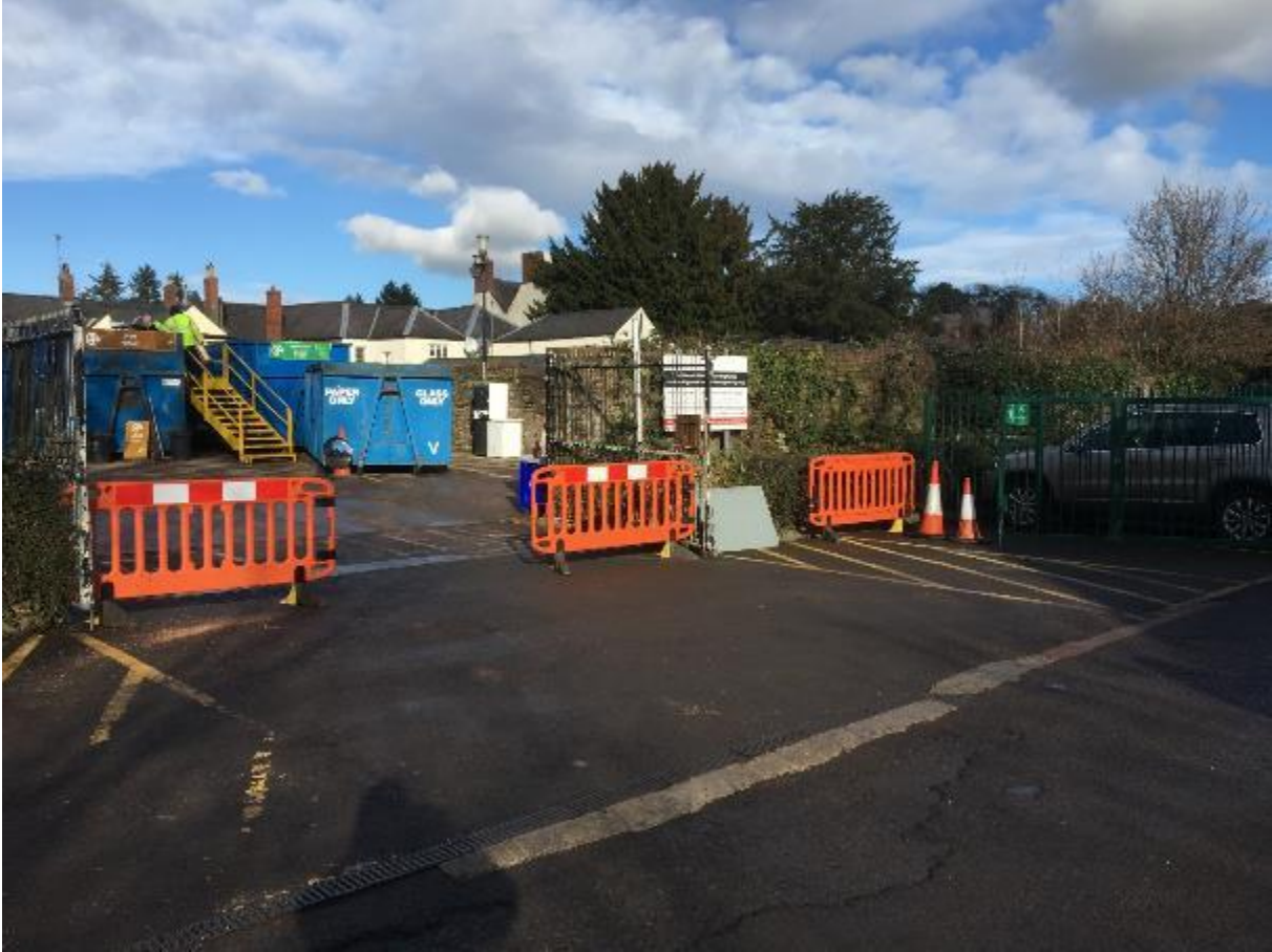
Figure 28: Usk Site Pedestrian Access to the Permitted Area
